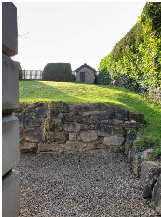
View from the west corner of 4 Greenroyd Court showing 3m elevation to top of garden and neighbours hedge.
